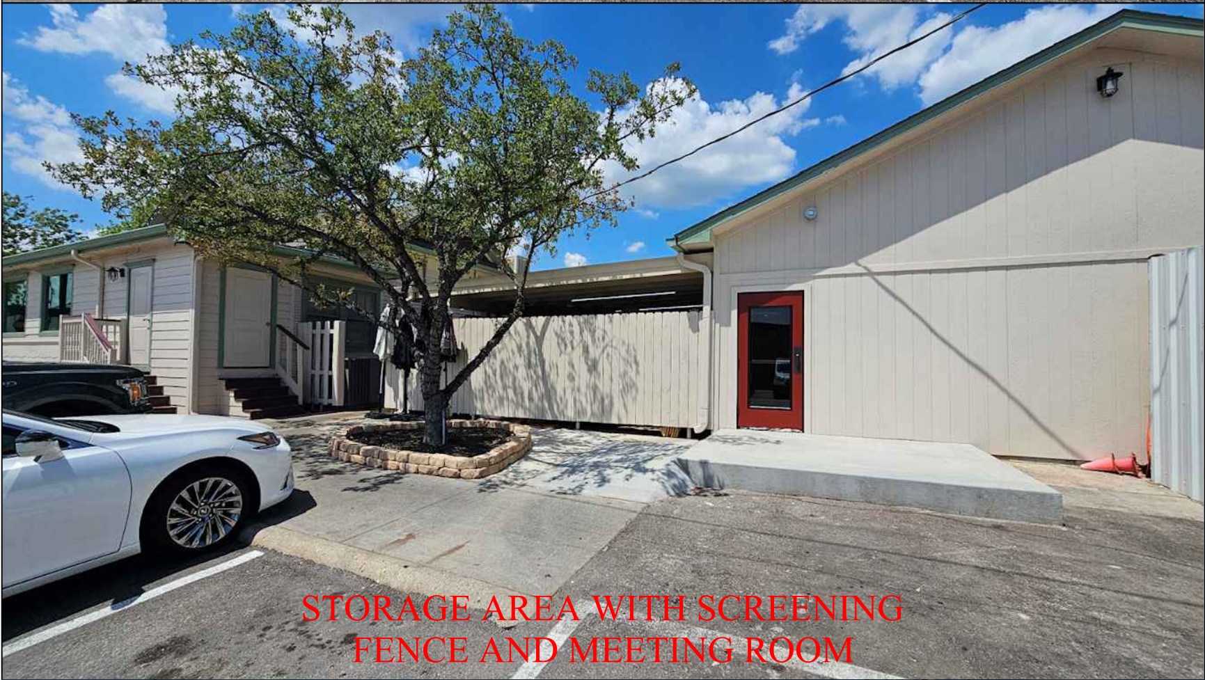
STORAGE AREA WITH SCREENING FENCE AND MEETING ROOM
