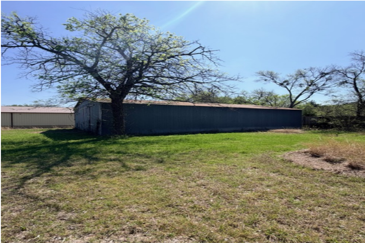
Exterior View – Side Elevation
