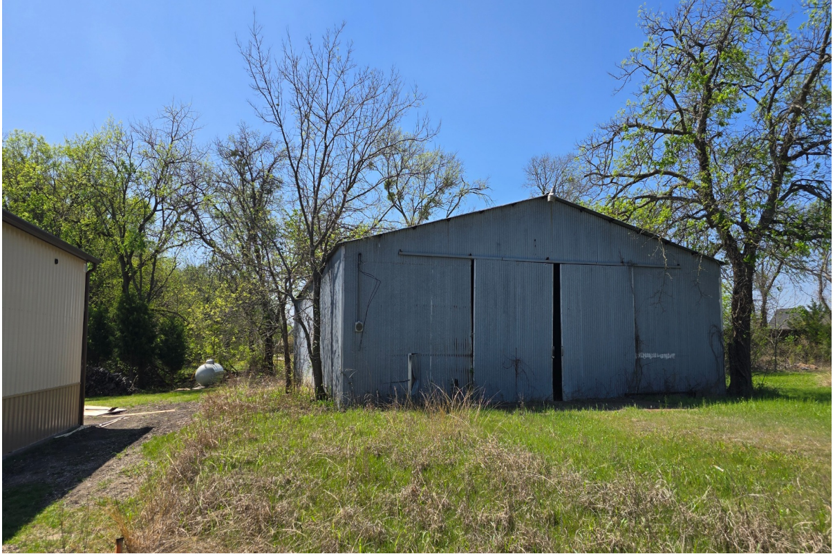
Exterior View – Overall Structure
