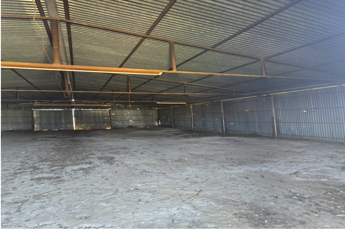
Interior View – Structure Condition
