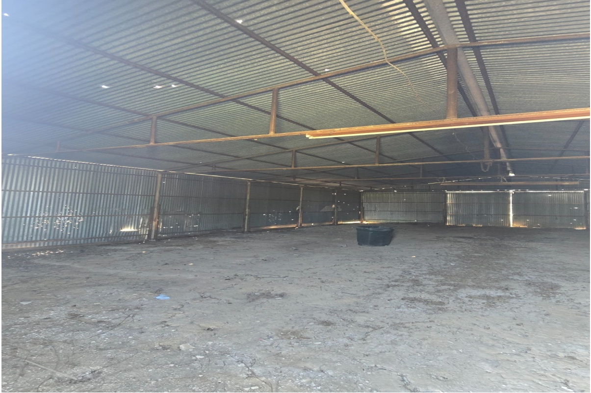
Interior View – Roof and Framing
