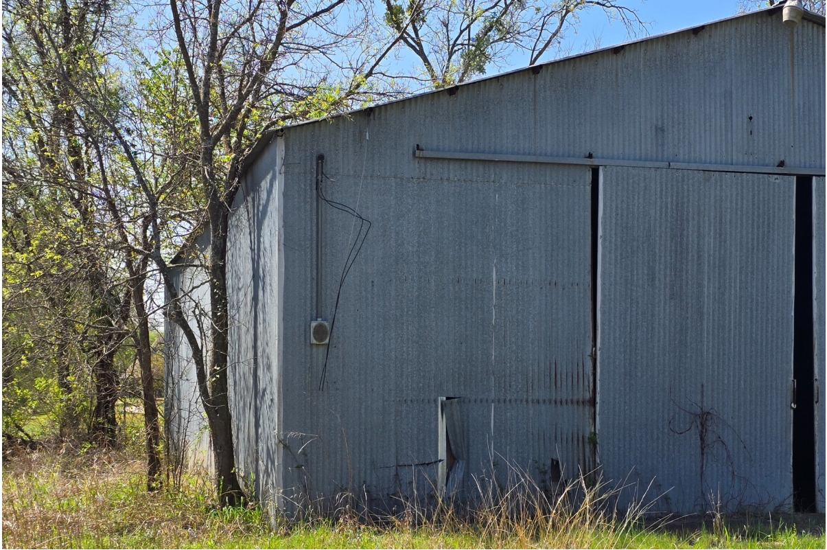
Exterior View – Rear/Side Condition
