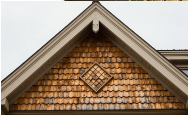
Wood Shingles / Shingle Patterns
