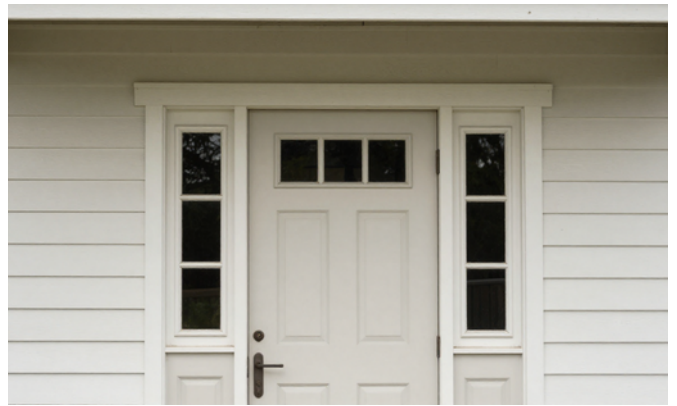
Simple Paneled Door with Glass Panes
