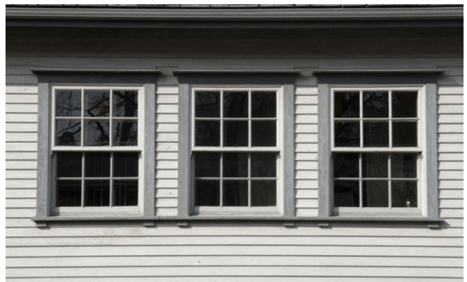
Banded Casement Windows
