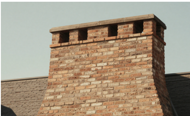
Low Massive Chimney
