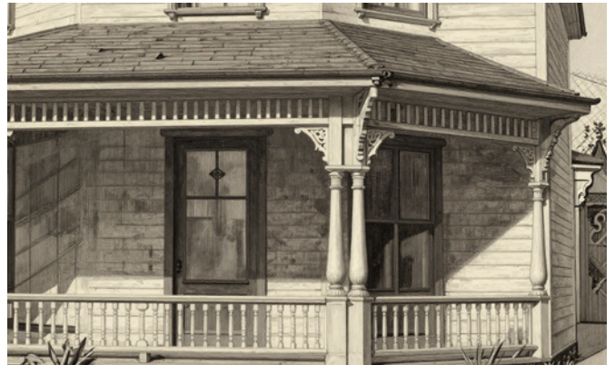
Entryway with Turned Posts
