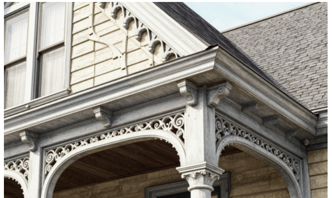
Carpenter Gothic Trim
