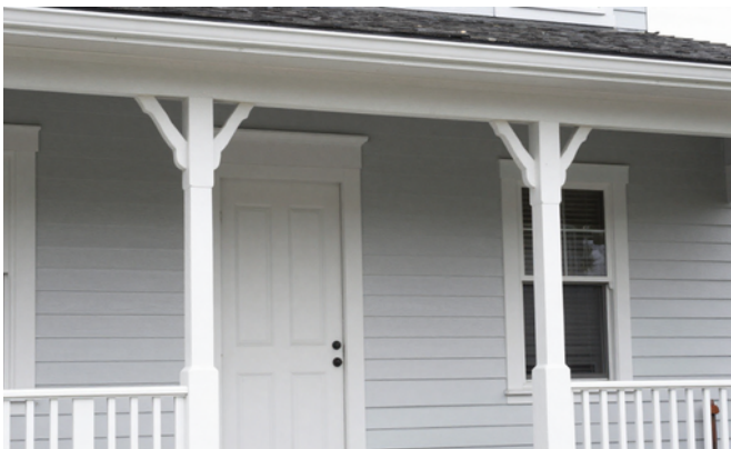
Front Porch with Tapered Supports
