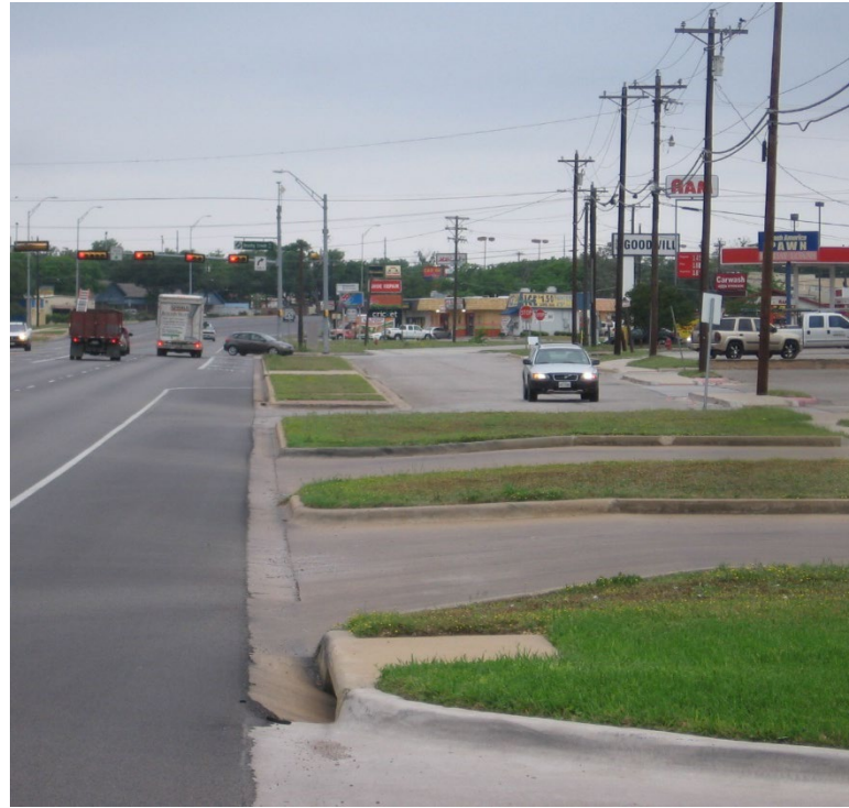
Example of Excessive Curb Cuts
