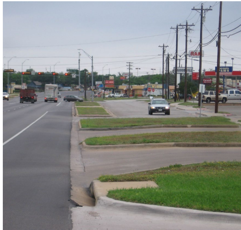
Example of Excessive Curb Cuts
