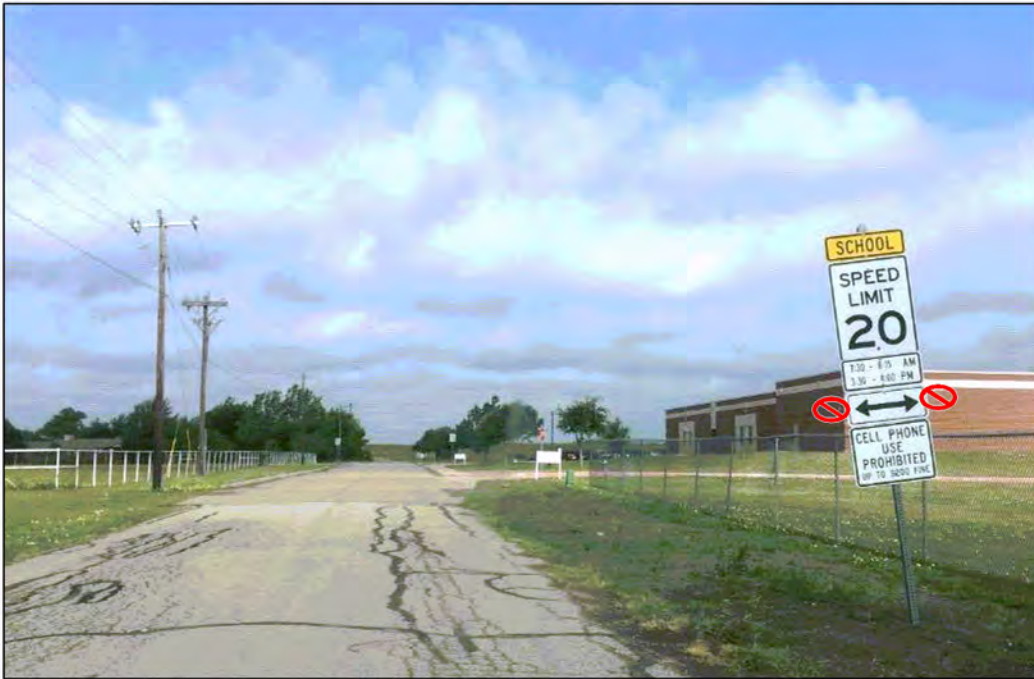
Figure 25: School Zone Sign Recommended Change on Westbound Old Hensley Lane
