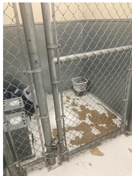
The flooring is peeling up and chain-link fencing is difficult to disinfect.
