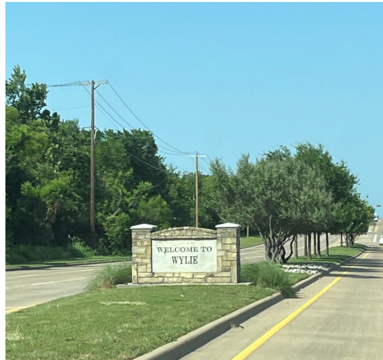
Existing Gateway Signage
