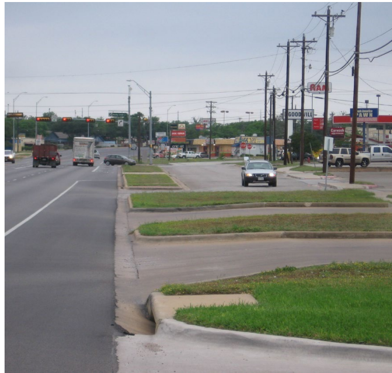
Example of Excessive Curb Cuts
