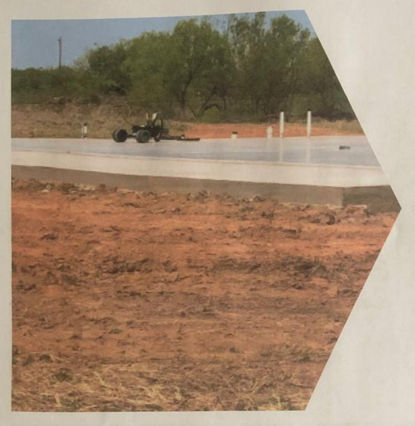
Concrete Slab Foundation
