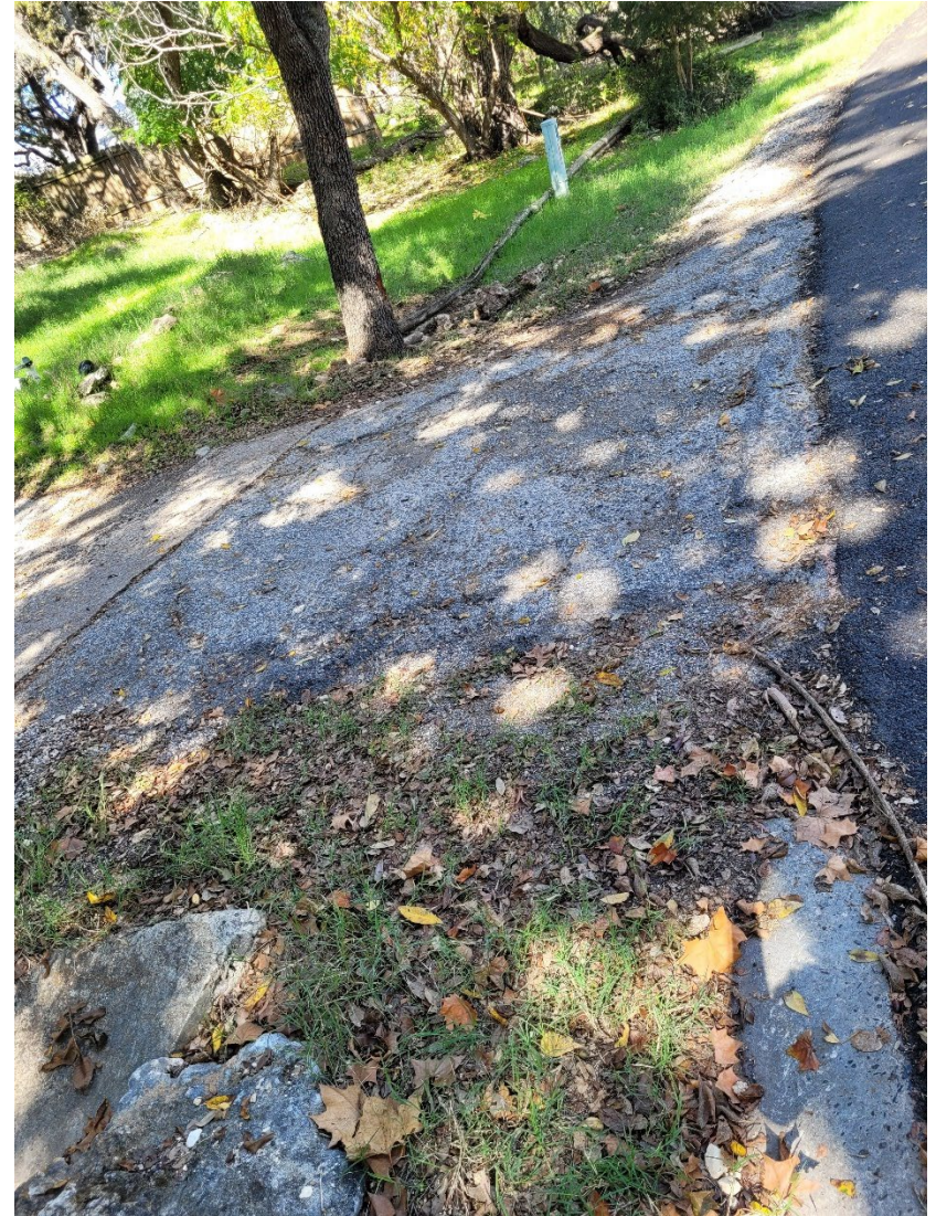
4 Tremont Trace – After (Asphalt Driveway & Approach)
