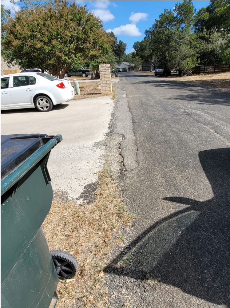
2023 Roads Project – Long and Short Driveways
