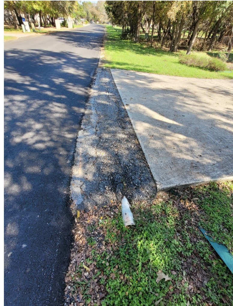
1 Woodview Court (Off of Canyon Creek Drive) – After
