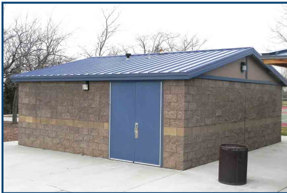
ST-6 Model attached to Restroom
