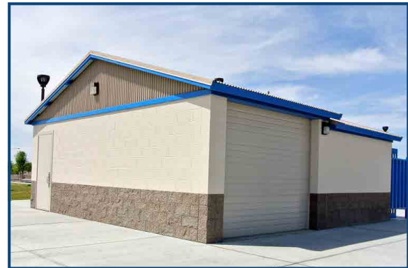
ST-10 Model attached to Restroom
