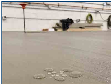
4 | Finished Slab of Specialized Moisture Resistant Concrete
