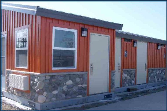
Laundry Room + Restrooms
