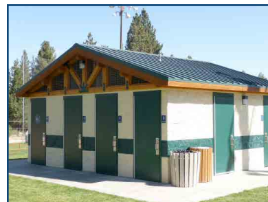
11 | Finished Building & Ready to Go! (literally)
