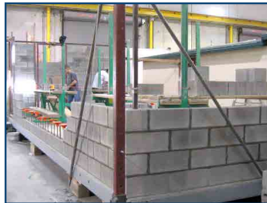
5 | CMU Walls Constructed on Concrete Slab
