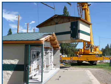
10 | Drop-In-Place Installation with a Crane
