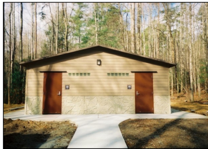
Men/Women ADA Restroom and Rear Showers
