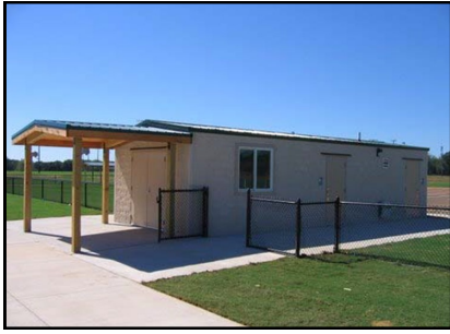
14' x 36' Restroom & Concession Facility
