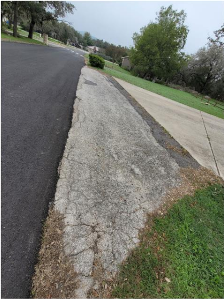
2023 Roads Project – Driveway Approaches
