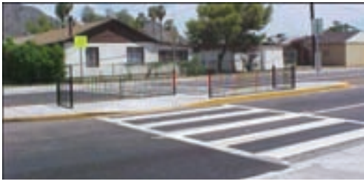
Two-stage crosswalks with fencing help direct pedestrians to look for vehicles coming from the right.
