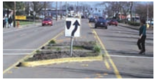
Pedestrian crossing islands provide a refuge when crossing wider roads.
