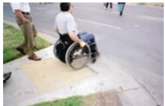
Well-designed curb ramps provide pedestrians with disabilities better access to the sidewalk system.
