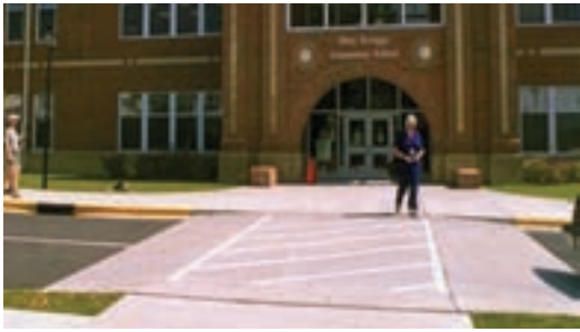
Traffic calming devices such as this raised crosswalk help illuminate pedestrian crossings and slow motor vehicle traffic.
