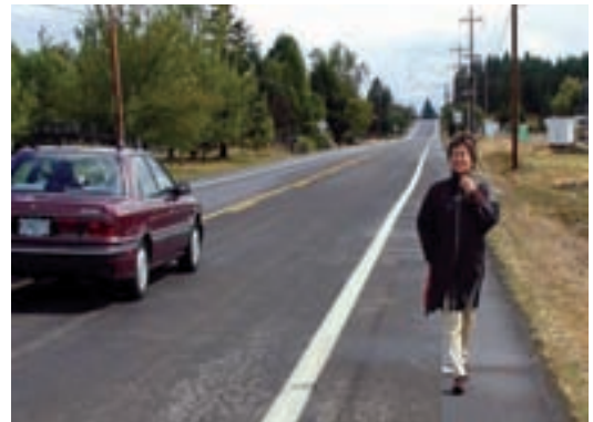
Paved shoulders offer pedestrians on rural roadways a safer place to walk.
