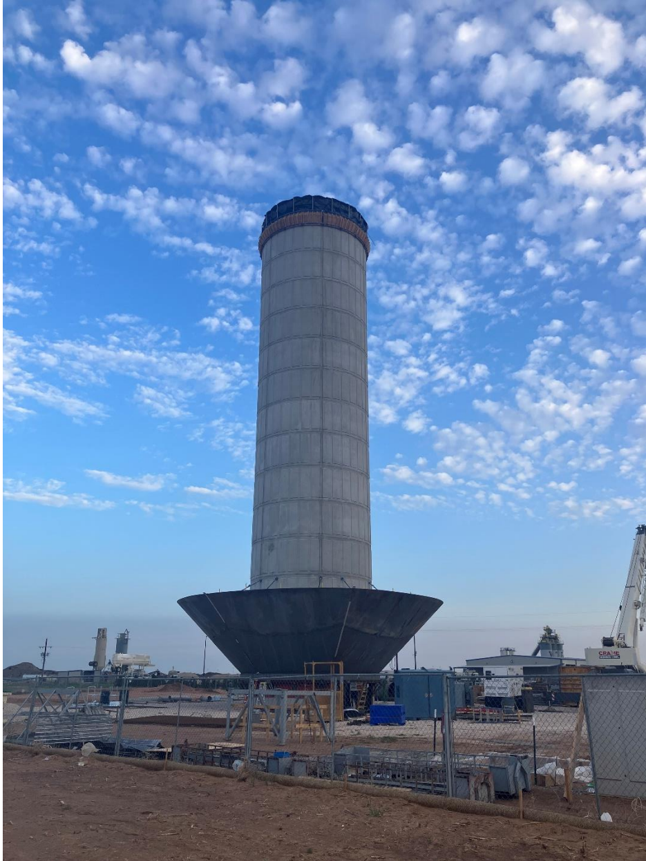
Tank Progress Photos
