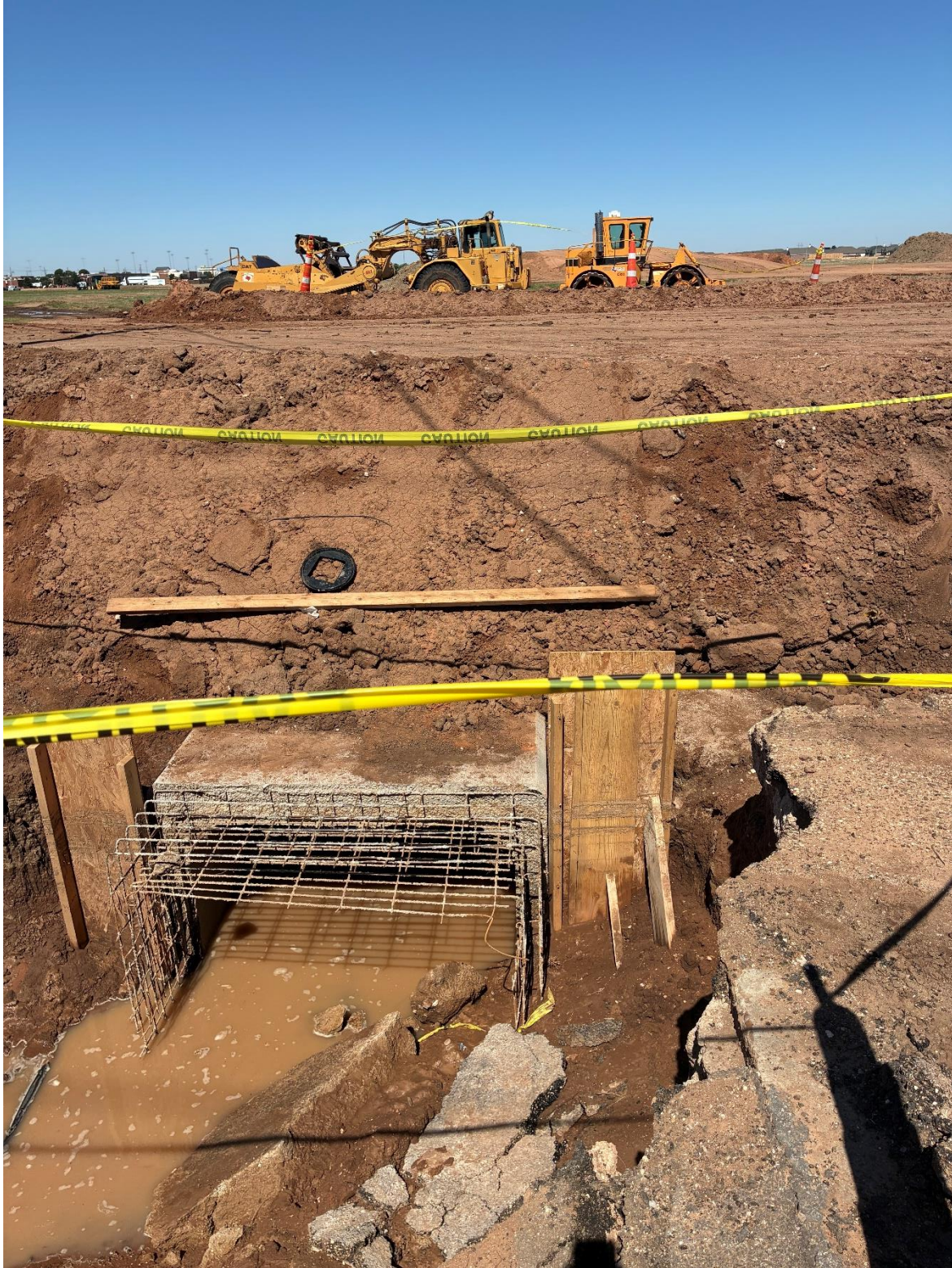
Alcove Progress Photos
