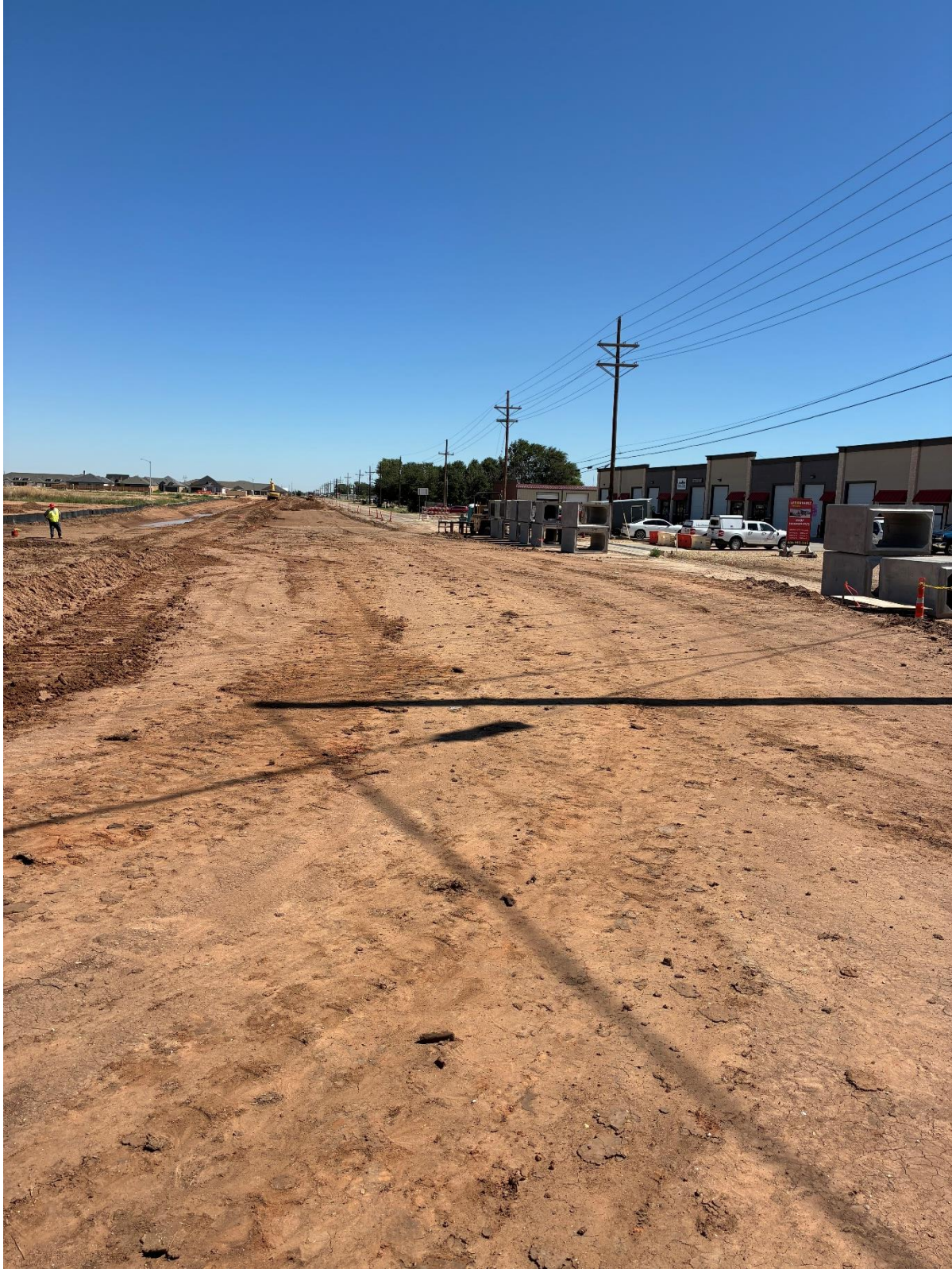
Alcove Progress Photos
