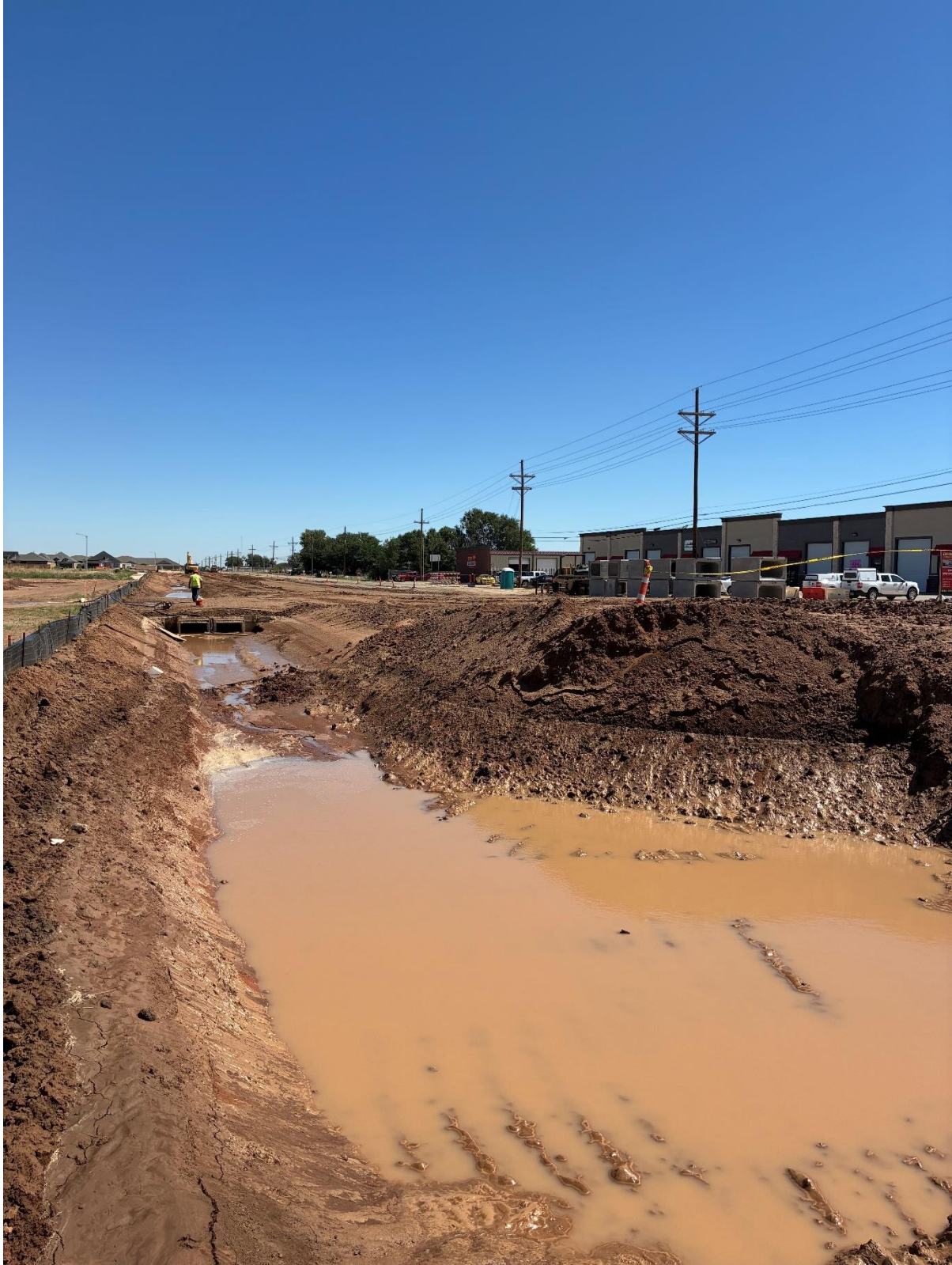
Alcove Progress Photos
