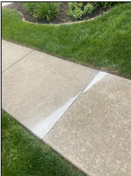
Sample Repair Photo: Defect 7 repaired on 05/19/25 at 507 Dickerson Dr. at 11:16 AM
