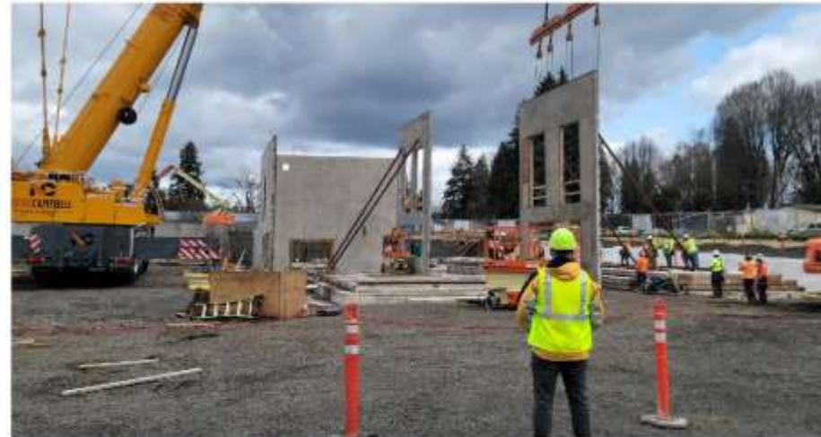
Wilsonville Public Works Complex 7
