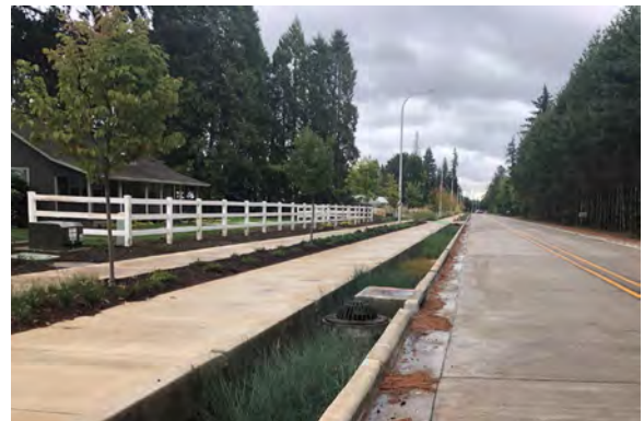
FIGURE 6: RECENTLY BUILT SIDEWALK AND CYCLE TRACK (EAST SIDE)
