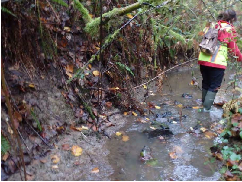
Photo 14 Channel with steep and eroding banks, and rock in channel
