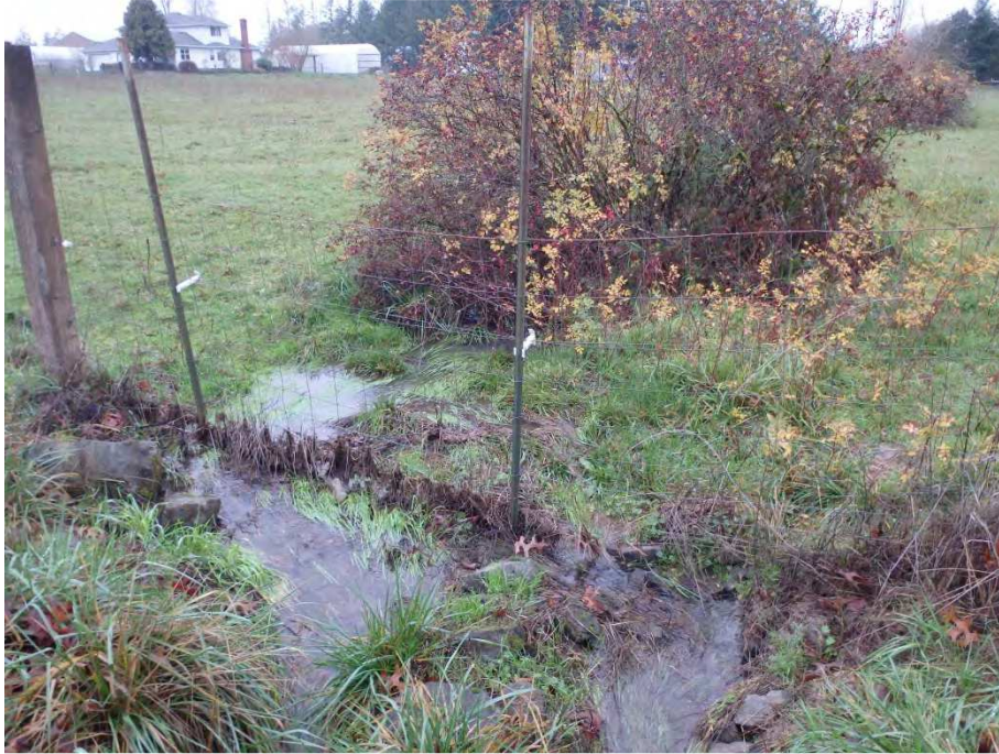
Photo 1 Channel in ROW on Frog Property
