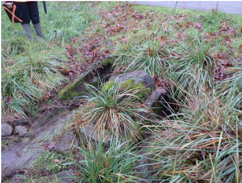
Photo 2 Upstream Ends of Culverts
