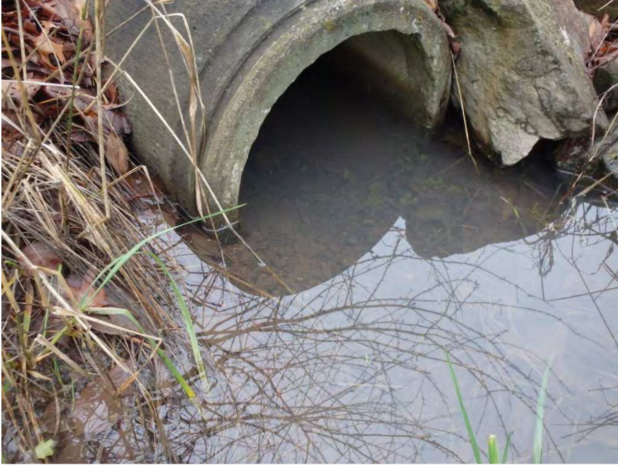
Photo 3 Downstream of culvert with gravel accumulation
