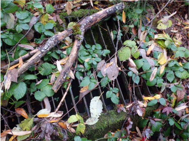
Photo 8 36-inch Outfall into Concrete Box
