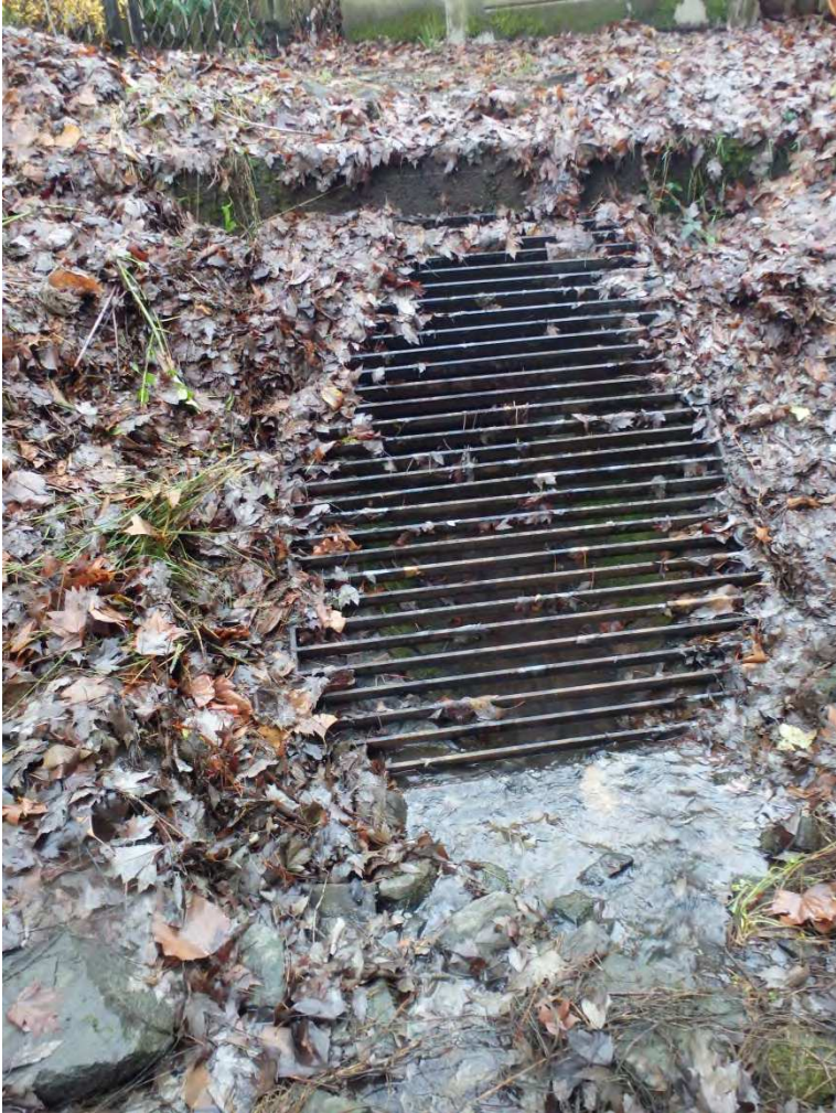
Photo 7 36-inch culvert under SW Willow Creek Drive
