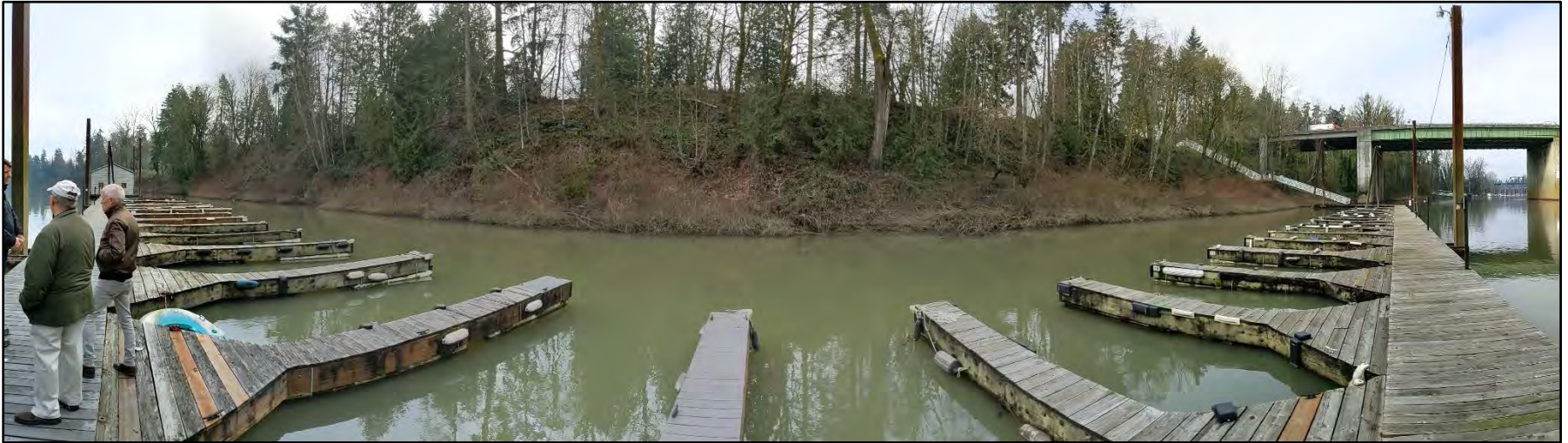
Photograph B-3. Panoramic photograph of the existing conditions within the SROZ and WRG looking east (left) and west (right). Dock to be replaced visible in the foreground. OHWL is apparent on bridge and dock pilings and along bank of the Willamette River.
