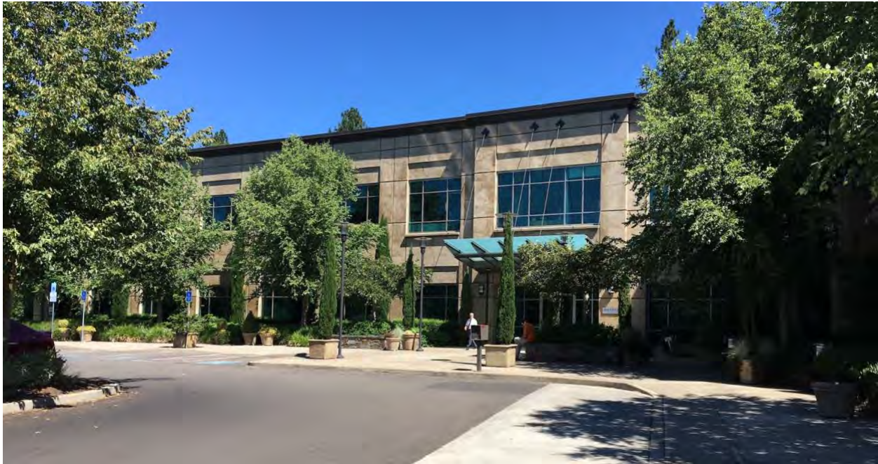
W1 in Wilsonville from 2009 at the front entry showing the simple palette of stained precast concrete walls, deep facade rustication with deeply set windows and extensive ornamental landscaping in addition to the preserved natural areas. This stain is in the warm range. Originally occupied by DWFRITZ Precision Automation until their expansion. Shell architecture by Lance Mueller & Associates (LMA).
