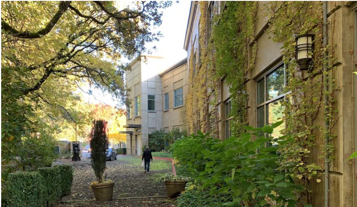
W1 in Wilsonville shown where it abuts an on-site SROZ natural area. This back-of-building view proves the high-quality materials and architecture extend all around the building. Vines on stained precast concrete walls are part of the architecture that include facade rustication and deeply set windows for visual interest. The big trees on left are part of the SROZ. Scale of this facade is similar to W5. Shell architecture by Lance Mueller & Associates. Address: 27200 SW Parkway Ave, Wilsonville, OR 97070
