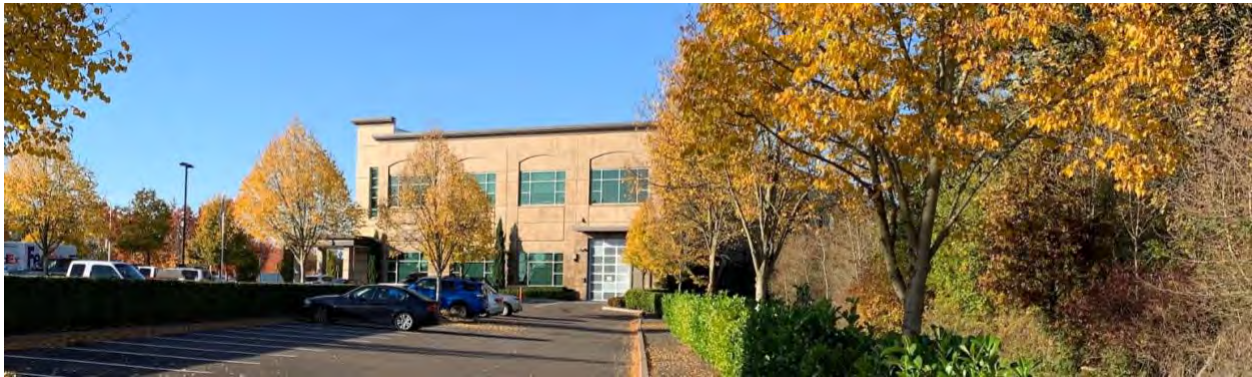
Two views of W3 in Wilsonville from 2012, the last part of the complex that includes W1 and W2 and borders the SROZ. Originally expansion space for DWFRITZ, it is now occupied by Sig Sauer, Electro-Optics. This wall stain is another warm example, and the warm afternoon sunlight is an influence. Shell architect is LMA. Address: 27100 SW Parkway Ave, Wilsonville, OR 97070
