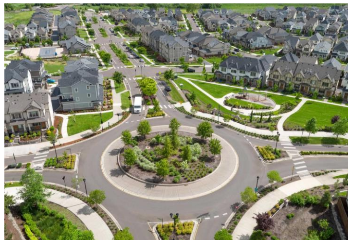
Wilsonville’s Villebois “urban village” development: Extensive infrastructure—including water, sewer, storm-water, roads, sidewalks, parks and other amenities—were funded with a combination of urban renewal (tax increment financing) and system development charges.
