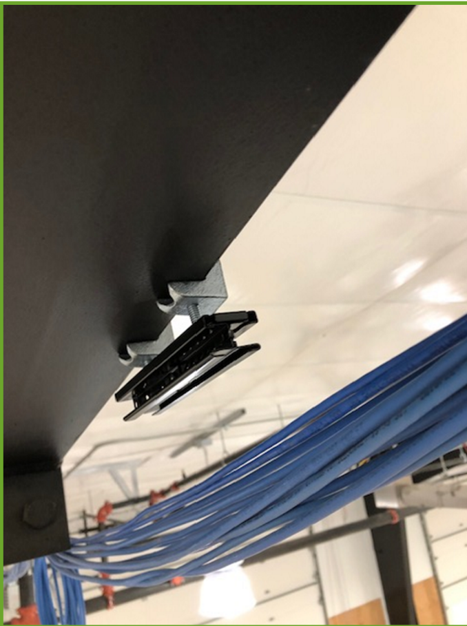
Custom bracket attached to support structure
