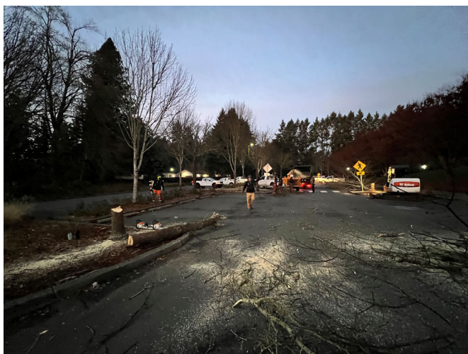
Tree Removal in Murase Plaza
