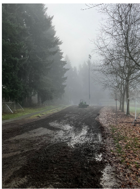
Grade work in Memorial Park
