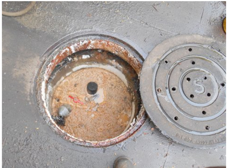
Grease in manhole
