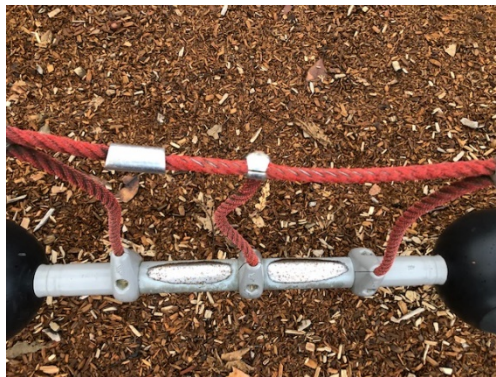
Braided cable exposed (high usage)
