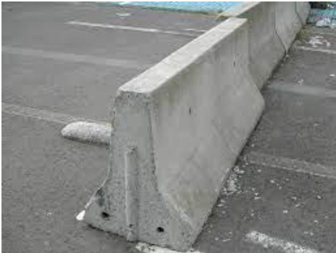
Example of Jersey Barrier
