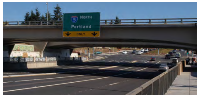
Looking east to the I-5/Wilsonville Road interchange.
