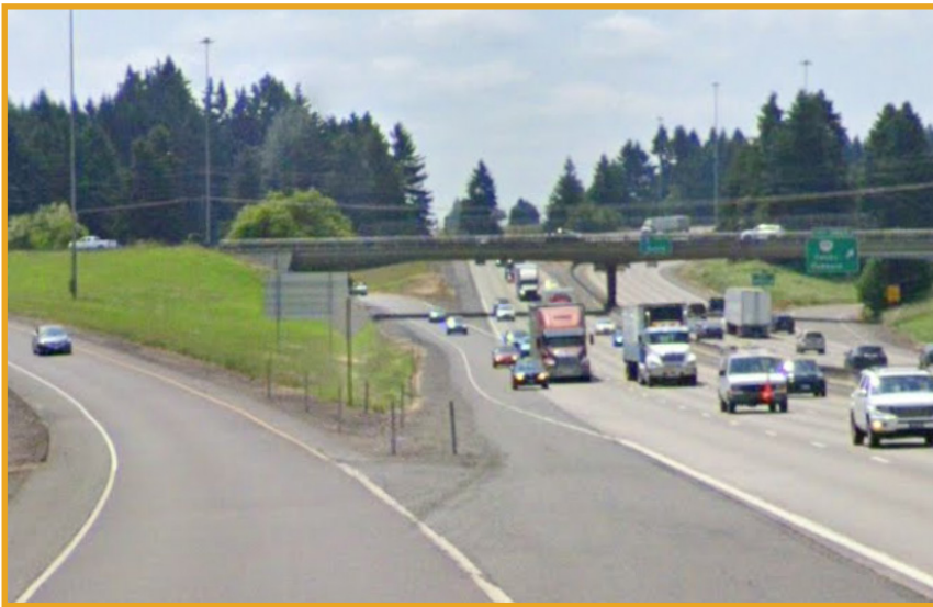
Above: Short merging distance between the OR 551 Canby-Hubbard entrance ramp and Charbonneau entrance ramp and heavy freight use cause safety conflicts resulting in a top 10% SPIS site.
