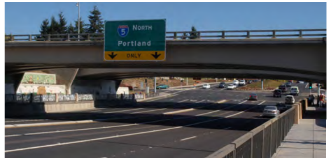
Looking east to the I-5/Wilsonville Road interchange.
