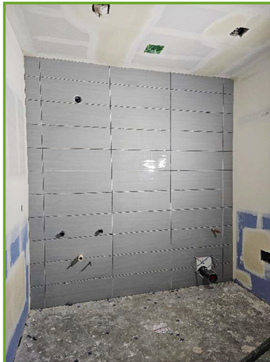
Tile in the reception area restroom
