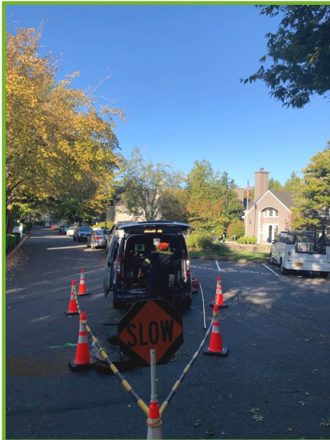
CCTV work in progress
