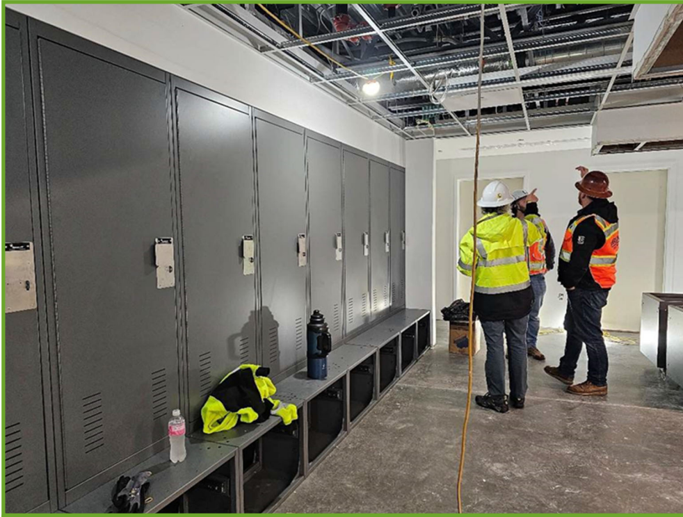
Locker room in the administration building
