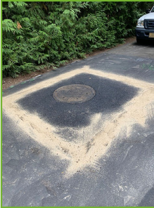
Manhole repair on Morey's Ct
