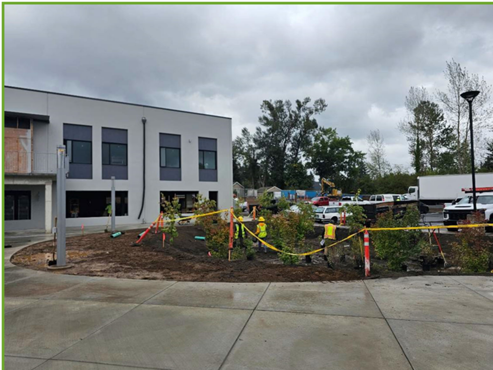
Planting of the water quality basin in the courtyard
