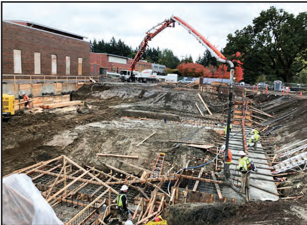
Pouring the footing for the Wilsonville High School Performing Arts Center expansion.
