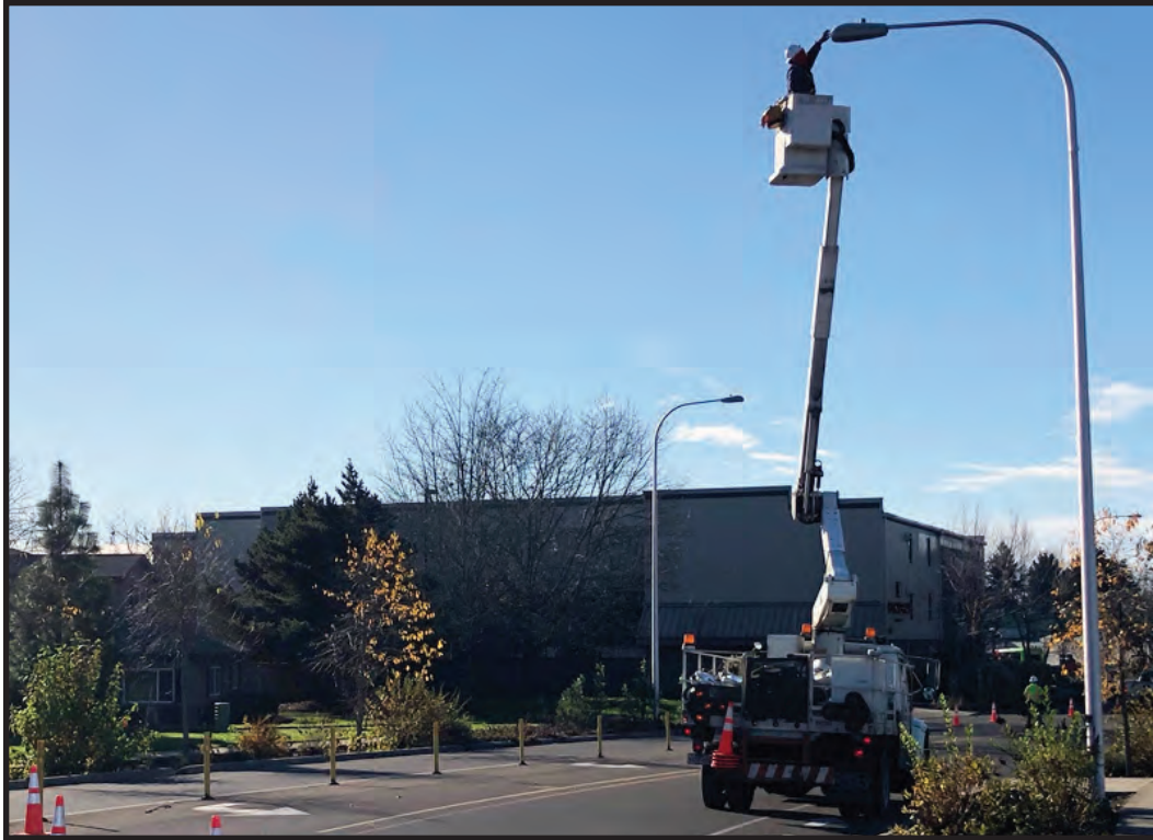
LED streetlight conversion project - light installation.
