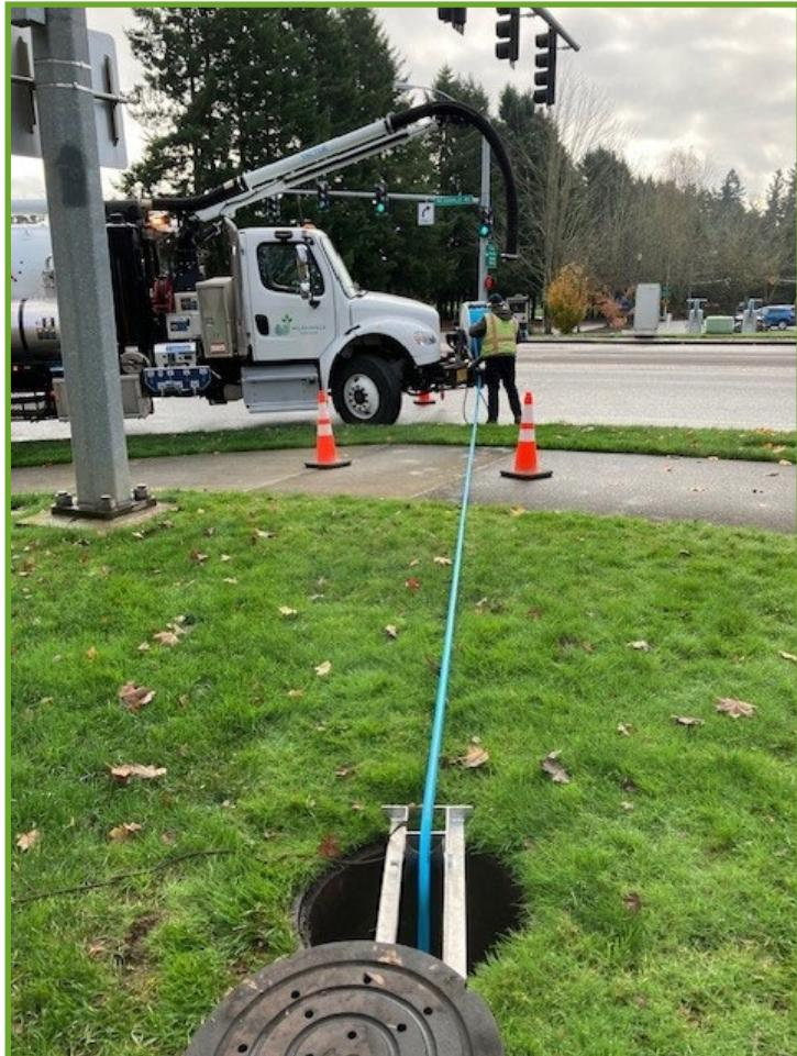
Video inspection of the pipes helps identify any problematic areas such as root intrusion or excessive debris collections.
