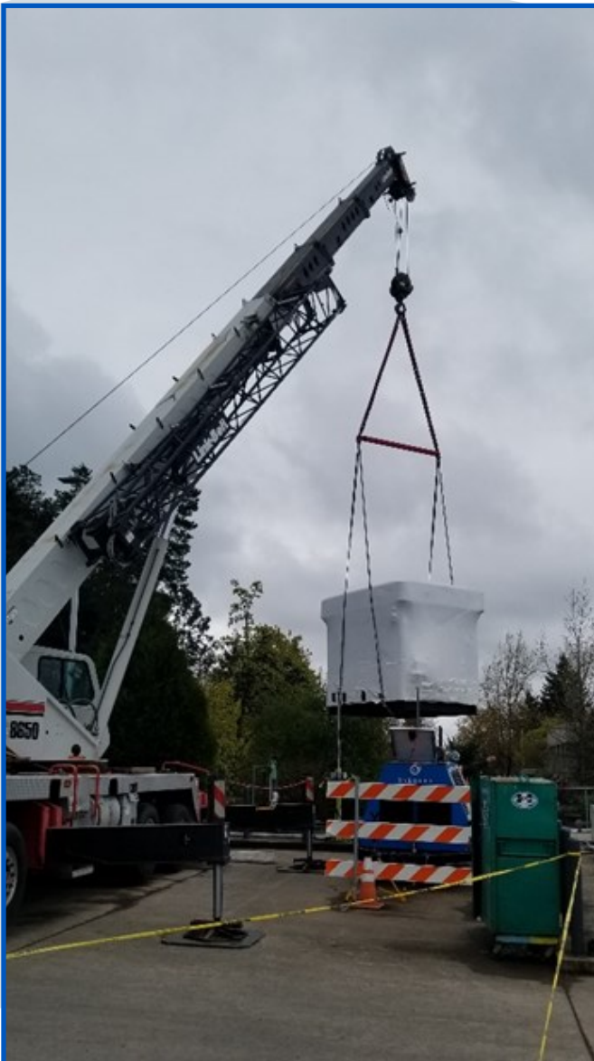
New compressor enclosure being set in place.
