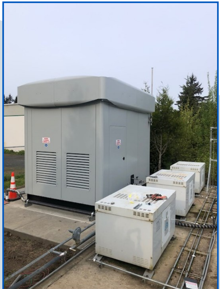
New compressor after installation.
