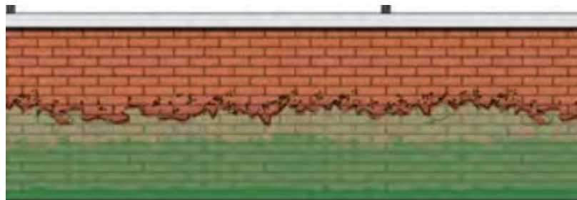
Figure X. 4 Foot Wall Along Stafford Road
