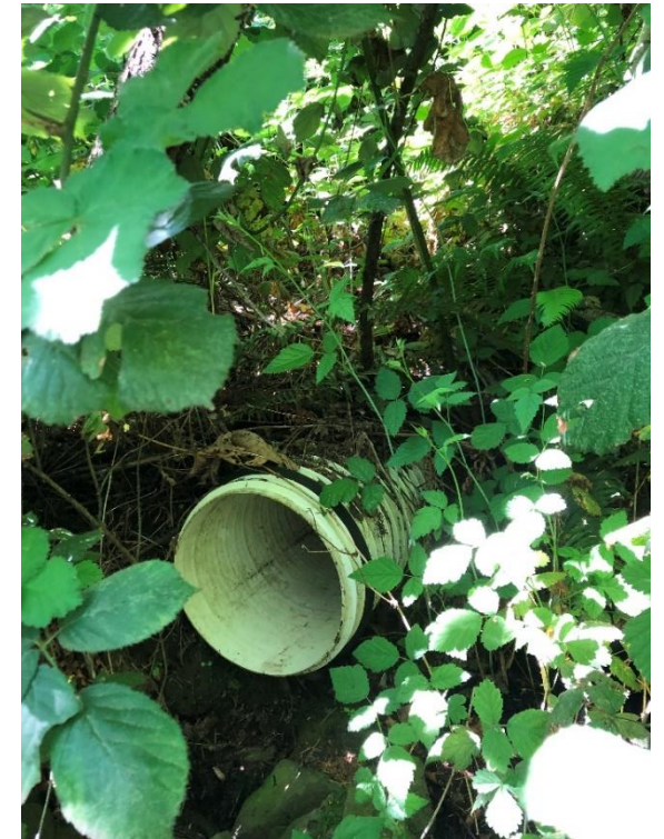
City-owned outfall pipe (May 2023)
