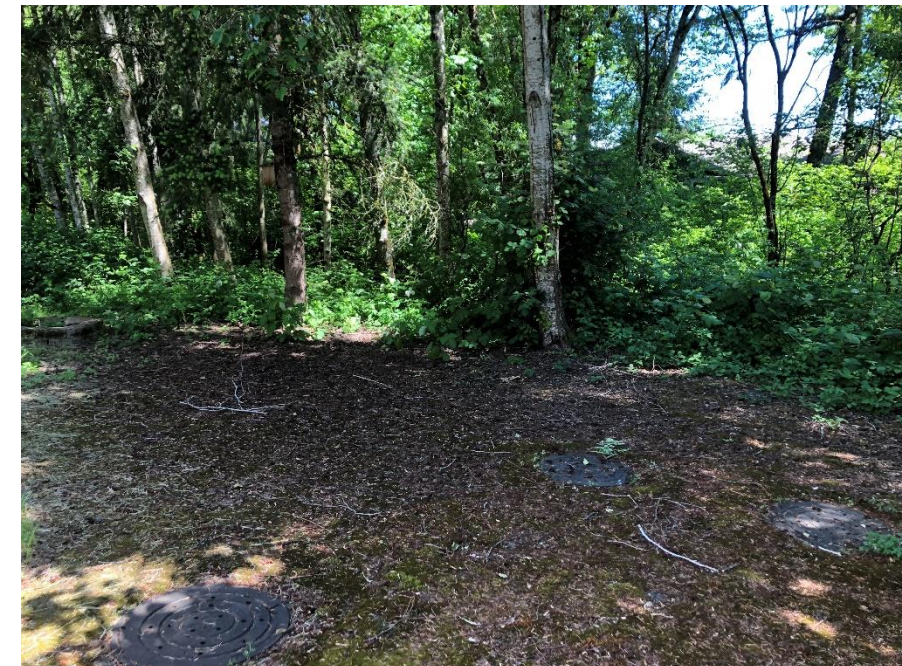
Upstream detention pipes location (May 2023)
