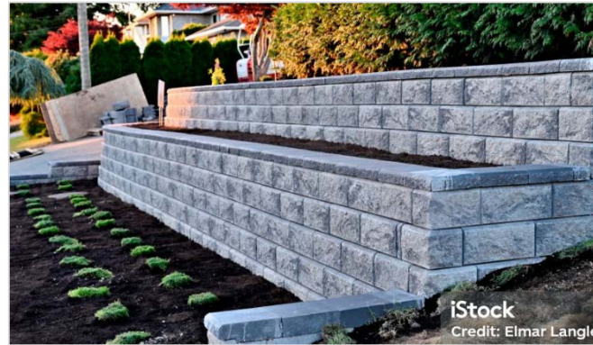
Tiered retaining wall with “horizontal offset” between lowest part and upper part(s) of wall
