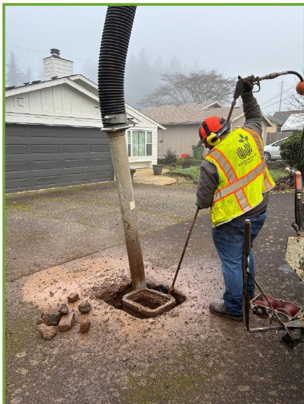
Some meters have been in the ground for as long as twenty years, and may be suffering from normal wear and tear. Replacing the older meters helps reduce the chances of equipment failure.
