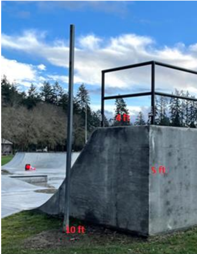
Wall 4 (side of wall 2)
