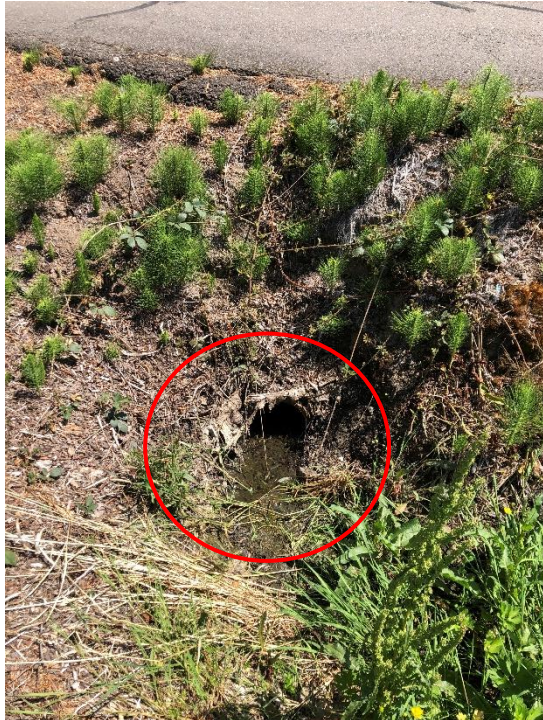
Culvert inlet under Rose Lane (May 2023)
