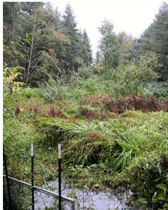
Dense, overgrown vegetation and accumulated sediment, combined with a lack of an outlet control structure, limits Library Pond's capacity and water quality function.
