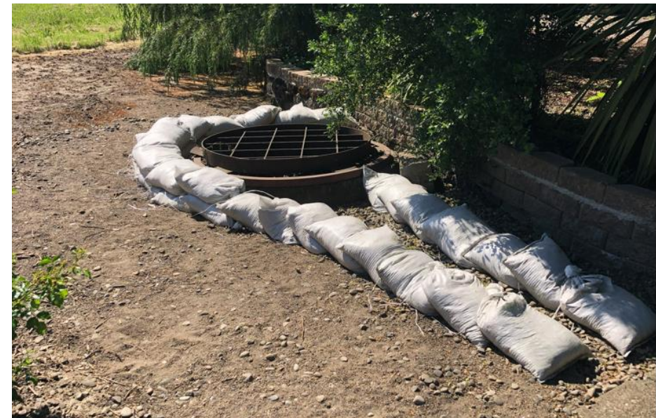
Existing Bubbler Structure (May 2023)
