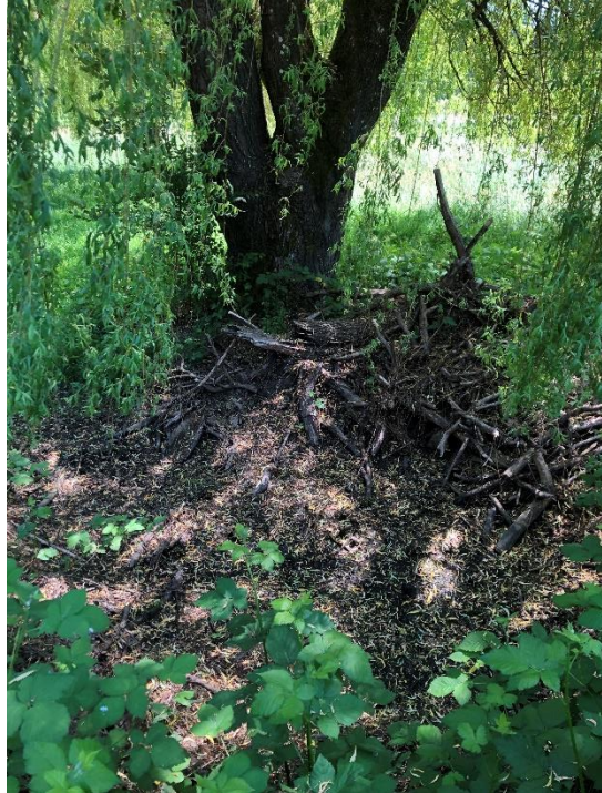
Downstream of culvert, east side of Rose Lane (May 2023)
