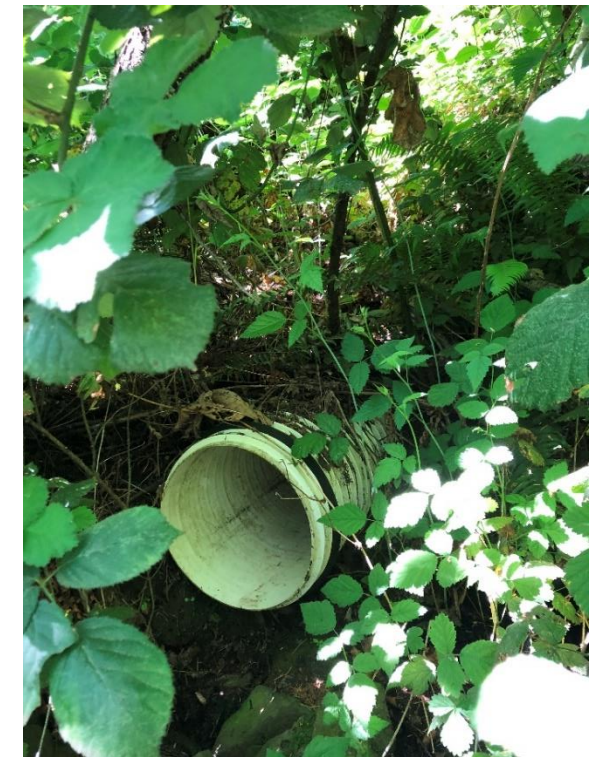
City-owned outfall pipe (May 2023)
