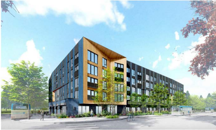
VIEW FROM NORTHEAST
