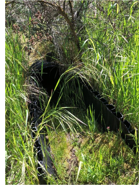
Garden Acres Pond Existing Inflow Pipe (May 2023)
