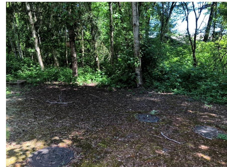
Upstream detention pipes location (May 2023)
