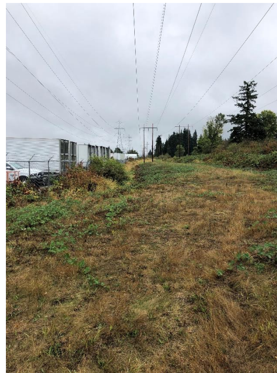
Wiedemann Ditch alignment (Sep 2021)
