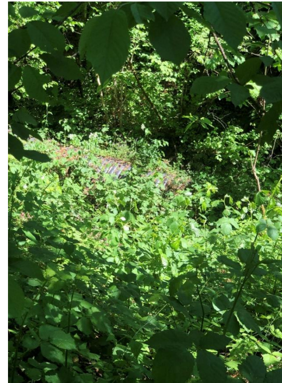
Streambank with resident-installed corrugated plastic pipe (May 2023)
