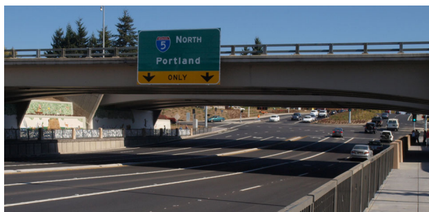
Looking east to the I-5/Wilsonville Road interchange.
