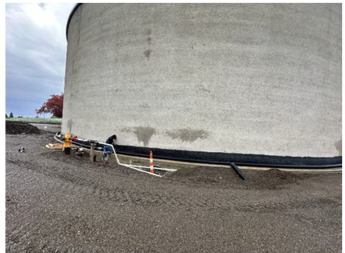
Waterproofing the tank exterior base
