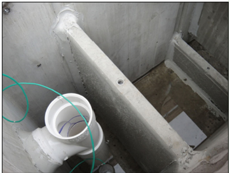
Oil separator vault—new replacement
