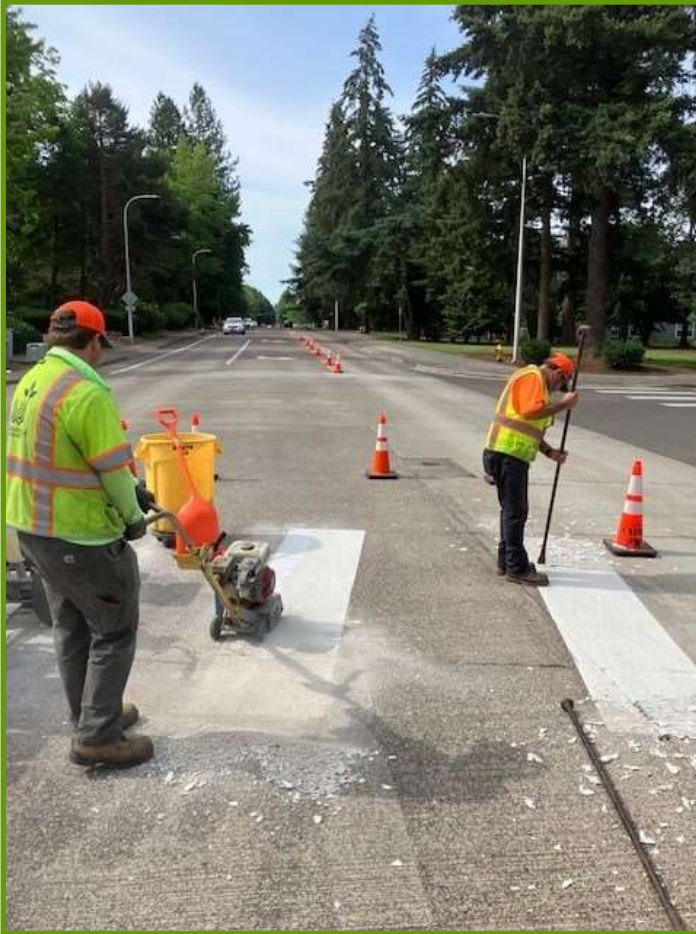
Crews are grinding out the existing striping using a grinder and pry bars where needed.
