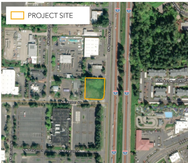
FIGURE 1: IONNA EV CHARGING STATION PROJECT SITE
