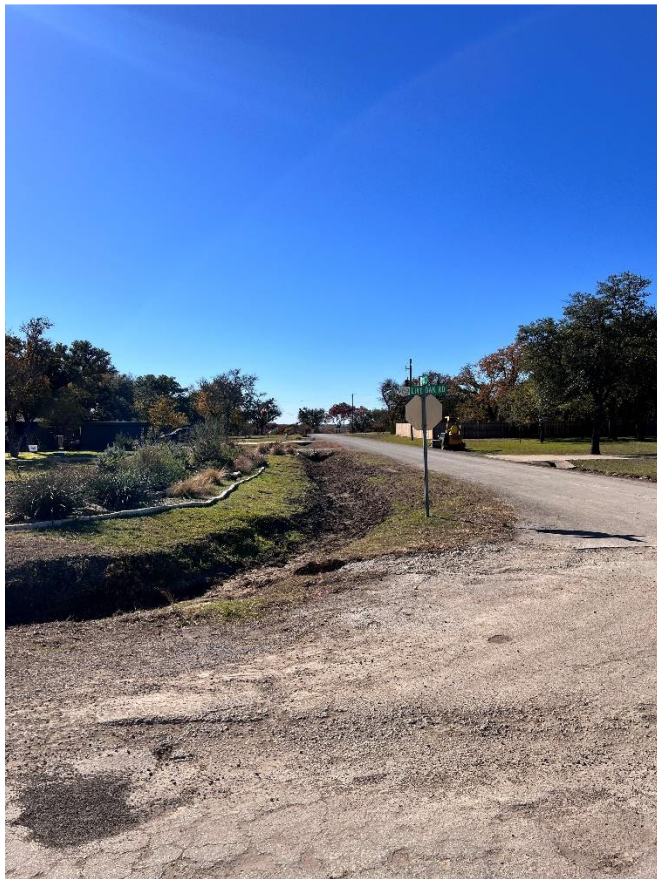
Channel B-1 looking south
