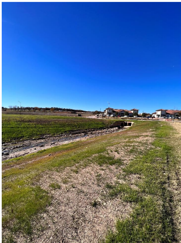
Channel C looking southwest
