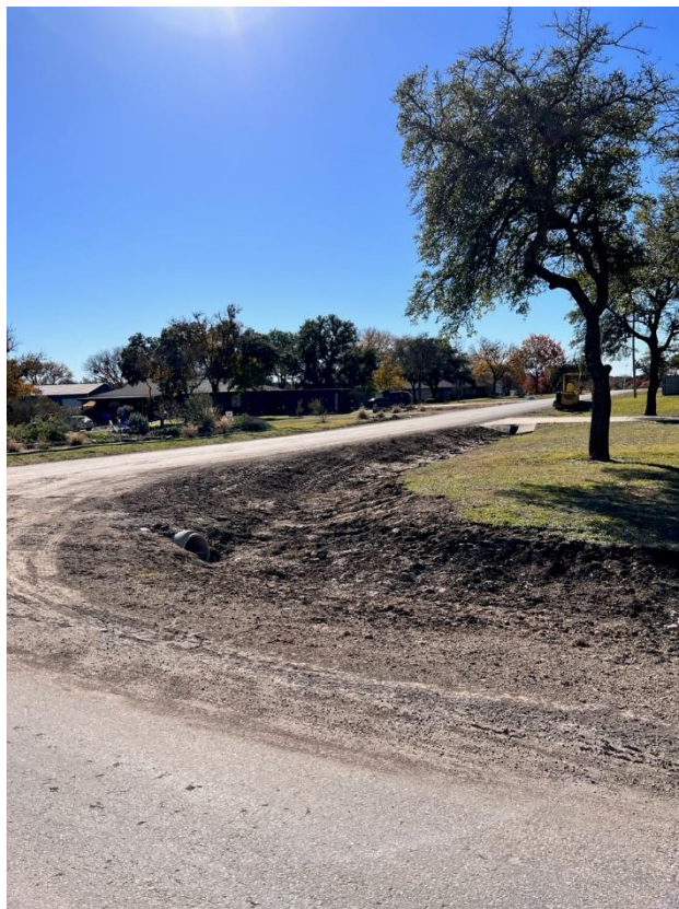
Channel B-2 looking southeast
