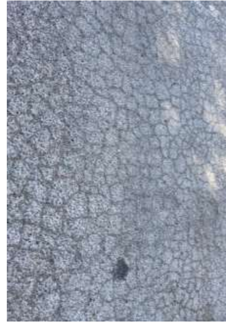
Alligator Cracks
