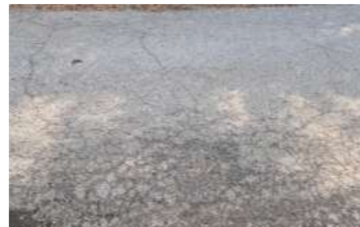
Block cracks
